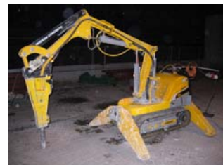
Night time shift, Brokk 90 with hydraulic breaker
