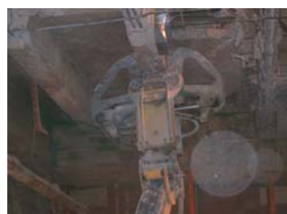
Daytime crushing, Brokk 90 with concrete crusher.
