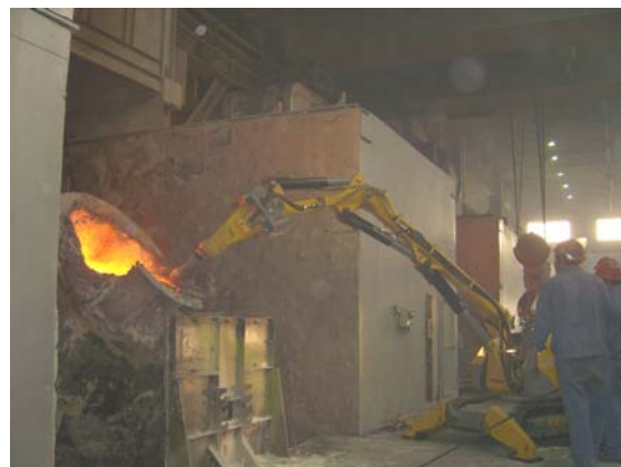
Cleaning of converter mouth with Brokk 330 in hot condition
