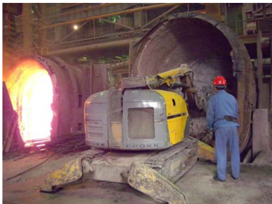
Safe and efficient ladle debricking
