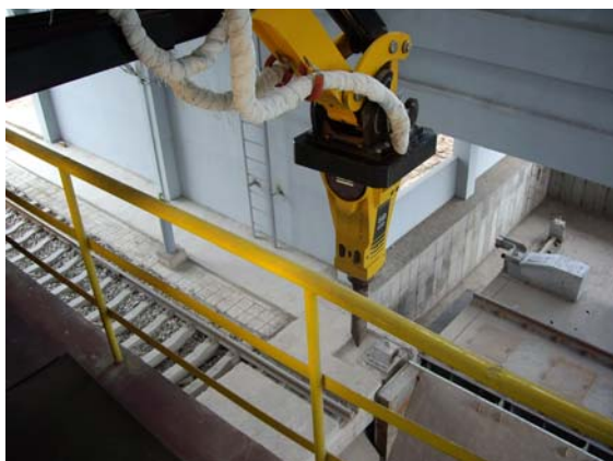
Brokk 330 used from a platform for cleaning of torpedoladle opening
