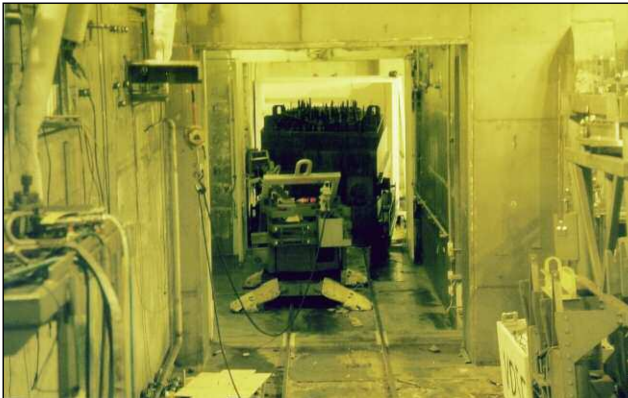
The melter encountered an interference on the tracks inside the transfer tunnel as it was being removed from the vitrification cell. The Brokk was used to position a jacking bar under the melter and return it to the tracks.
