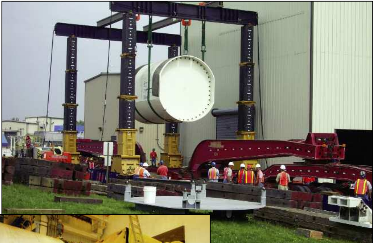
Top: The steel container constructed to hold the CFMT is unloaded from a truck upon arrival at the WVDP. It is elevated on a set of gantry cranes erected in front of the Load In/Load Out Facility to support the lifting and lowering of heavy containers removed during the dismantlement project.
