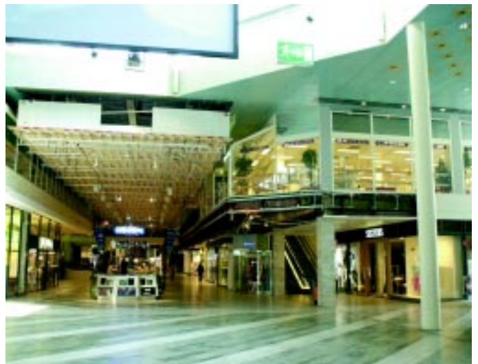
The renovation is divided in two different phases. During the first phase half the shopping centre will remain open to the public.
