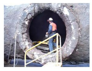
With this small but highly efficient machine, the job takes only 1 to 2 days compared to the original 6 to 10 days. At the same time, the number of accidents was reduced significantly. This increased efficiency of cleaning allows the plant to clean the torpedoes more frequently to further increase the productivity of the plant.
