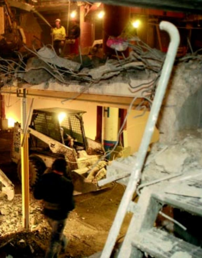
Six remote controlled demolition robots were used at the same time during the most intensive period of the project. The most sensitive parts of the demolition were carried out during night time and weekends to minimise the environmental problems.
