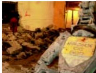
All the Brokk machines were equipped with silent demolition tools as this project was under special regulations concerning noise, dust and vibrations.
