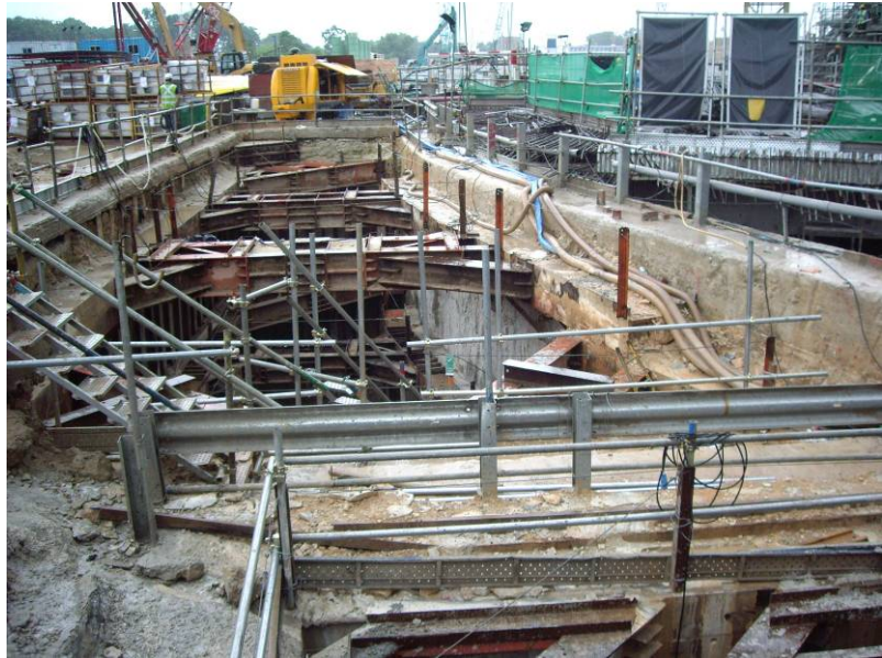
Two diaphragm walls with steel struts in between for stabilization
