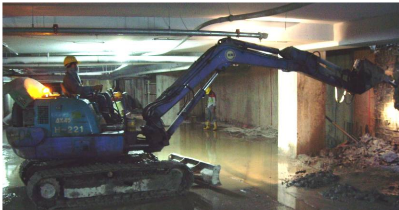
The mini-excavator's low-energy breaker with an arm-system optimized for digging resulted in a very low performance
