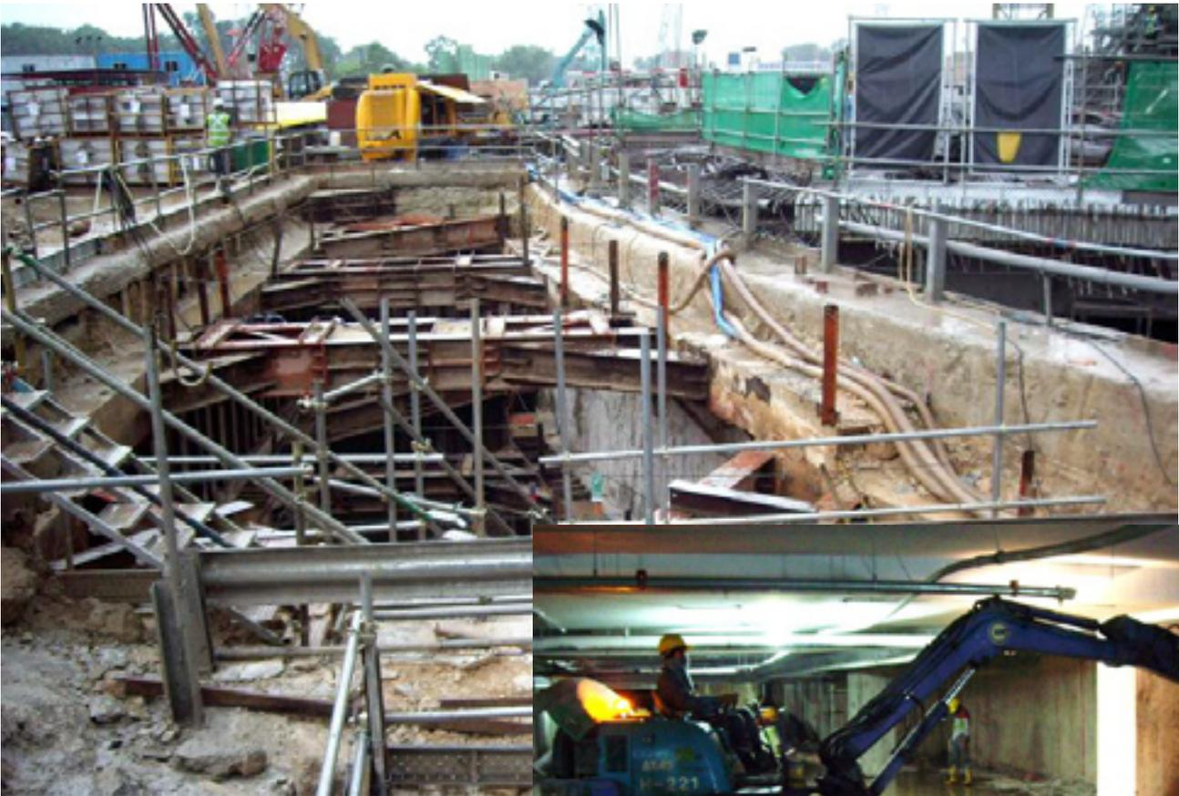
Two diaphragm walls with steel struts in between for stabilization
