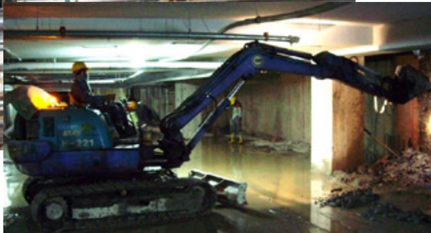
The mini excavator's low energy breaker with an arm system optimized for digging resulted in a very low performance
