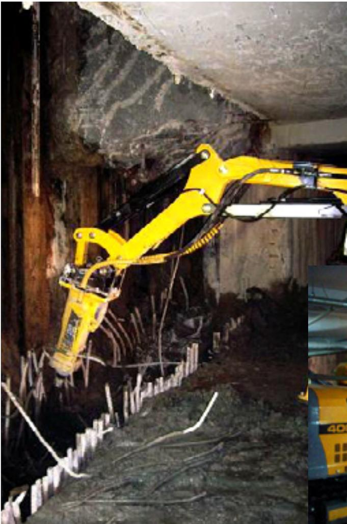
Brokk 400 breaking roughly 4 cubic meters per hour allowing for total removal of 36 cubic meters in 3 days.
